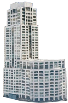
The Heritage at Trump Place 250 Riverside Boulevard
